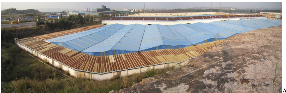
large licensed e-waste recycling plant located in an industrial park. Photo credit: Yvan Schulz
